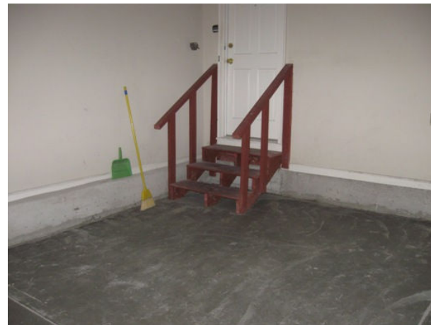
Next day the steps were replaced.
