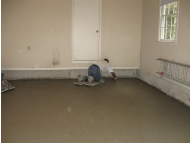
Hand troweling begins...
