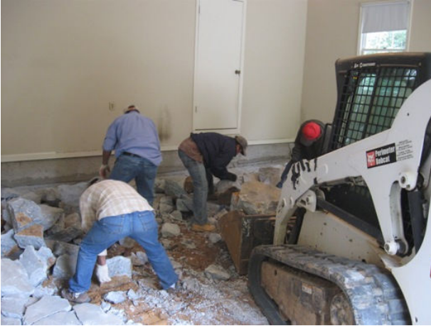
Remov- ing the old concrete.
