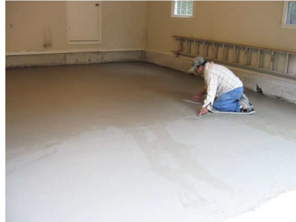
... three times using the knee skids ...
