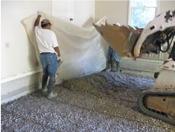
Carefully dumping the new concrete.
