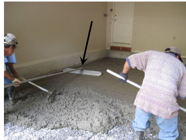
Starting to float the new concrete as more is being added.
