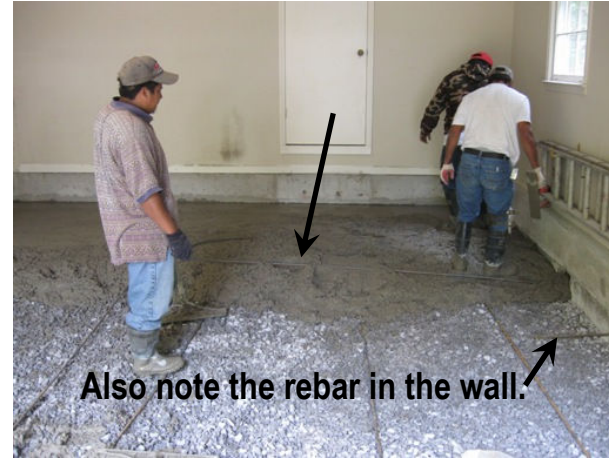
Perpendicular rebar being worked into the concrete.
