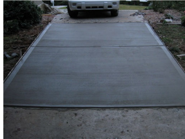
Finished driveway section.
