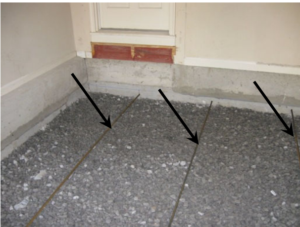
Some of the rebar added.
