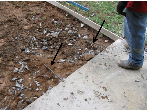
Rebar into existing concrete.
