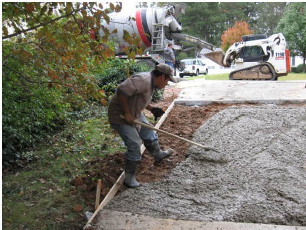
Working in new concrete.
