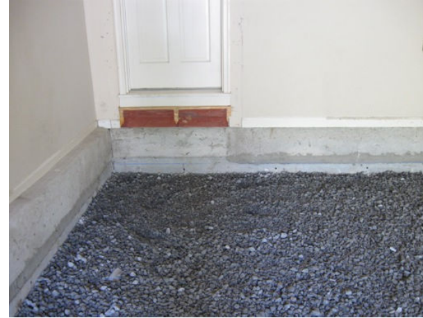
Crushed rock base.
