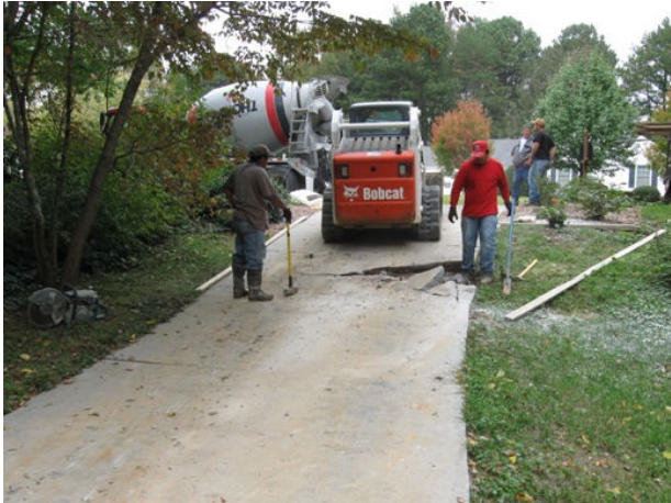
Old section being removed.
