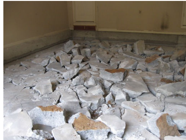
Old concrete all broken up.
