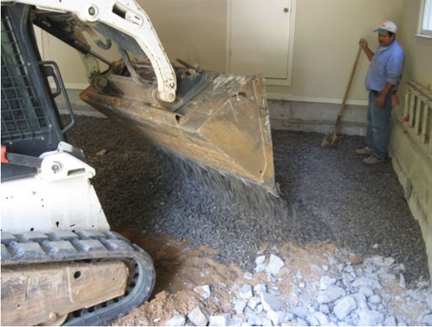
Adding crushed rock base.
