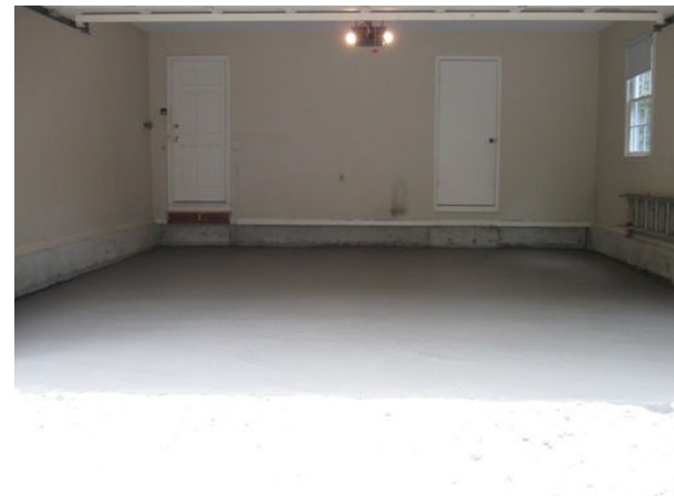
New garage floor ready for hand troweling.
