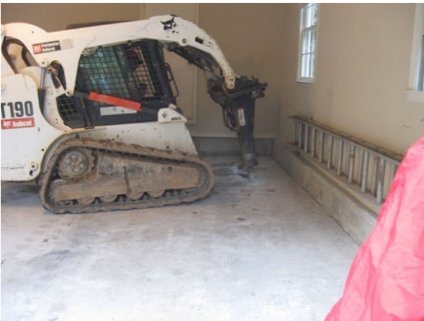
Jack hammering out the old concrete.
