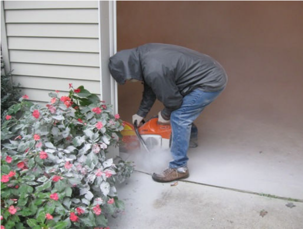
Cutting existing concrete.
