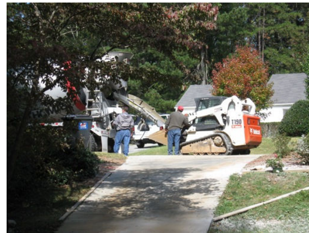
Concrete being loaded into the bobcat.
