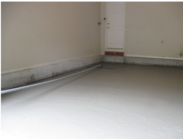
and the final floating of the floor.
