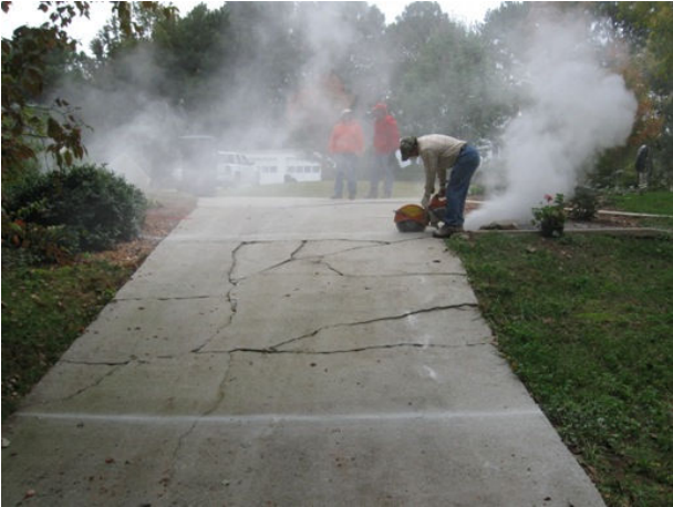
Cutting out driveway section.
